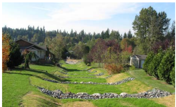
Vegetated swale after 2011 construction
