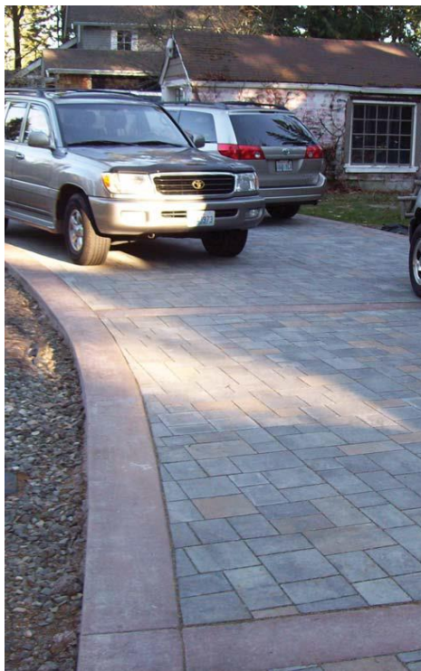
HIP permeable paver driveway in use. Installed 2013.
